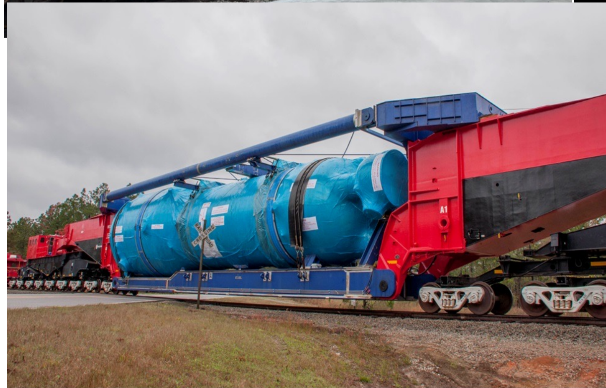
Vogtle Unit 3 steam generator B arrives at the Vogtle 3 and 4 construction site.
